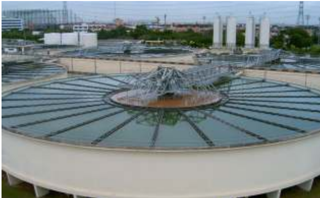
190 ft diameter HRSCC
