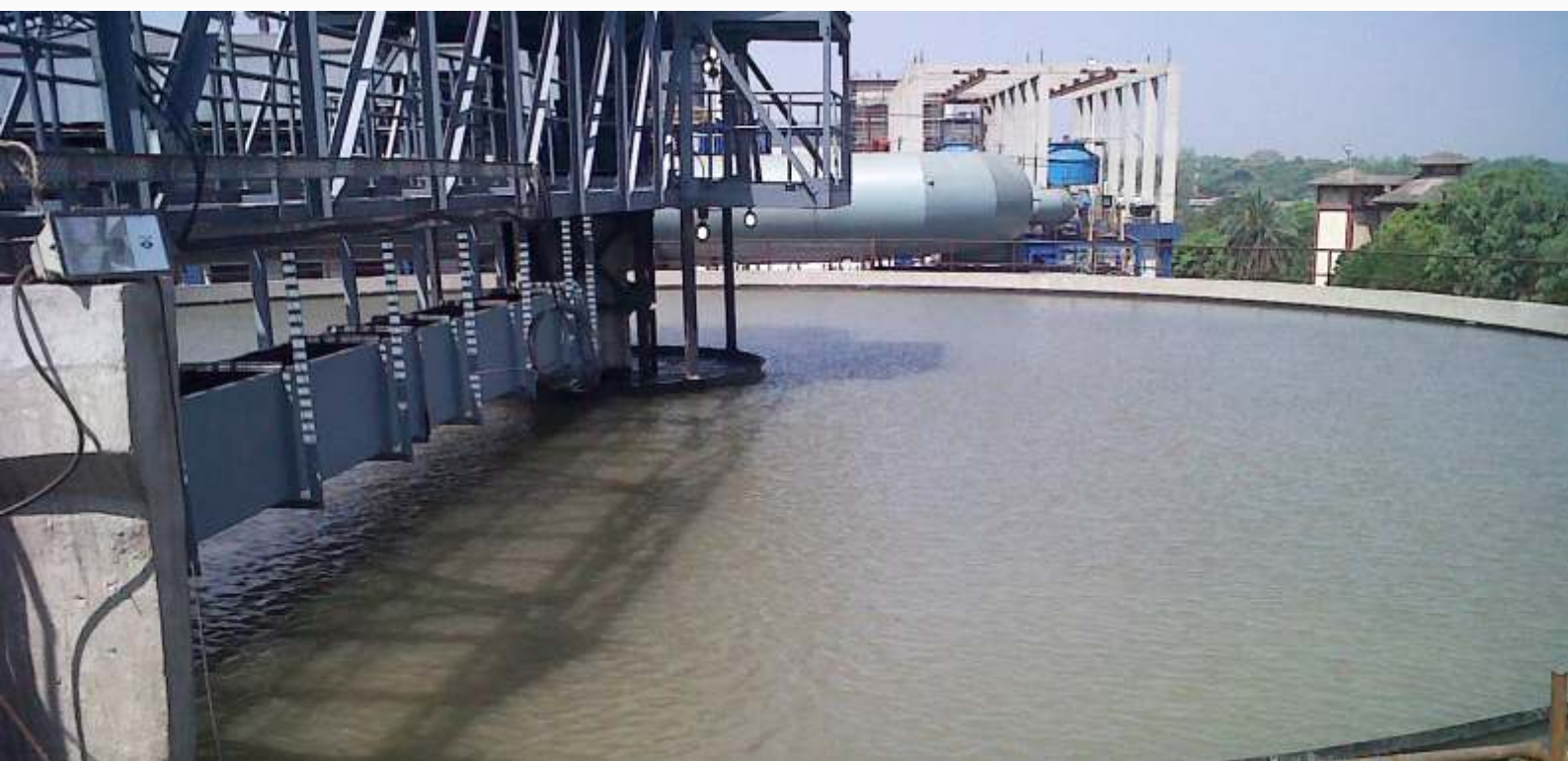
102 ft diameter high rate thickener with Hydraulic Drive and Hydraulic lift
